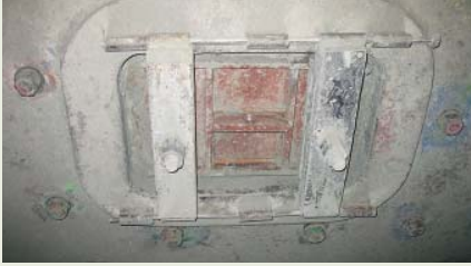
Mill maintenance access door
